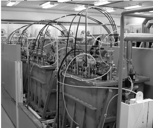
Figure 1: A view of ANU LINAC comprising twelve SLRs in four module cryostats.
